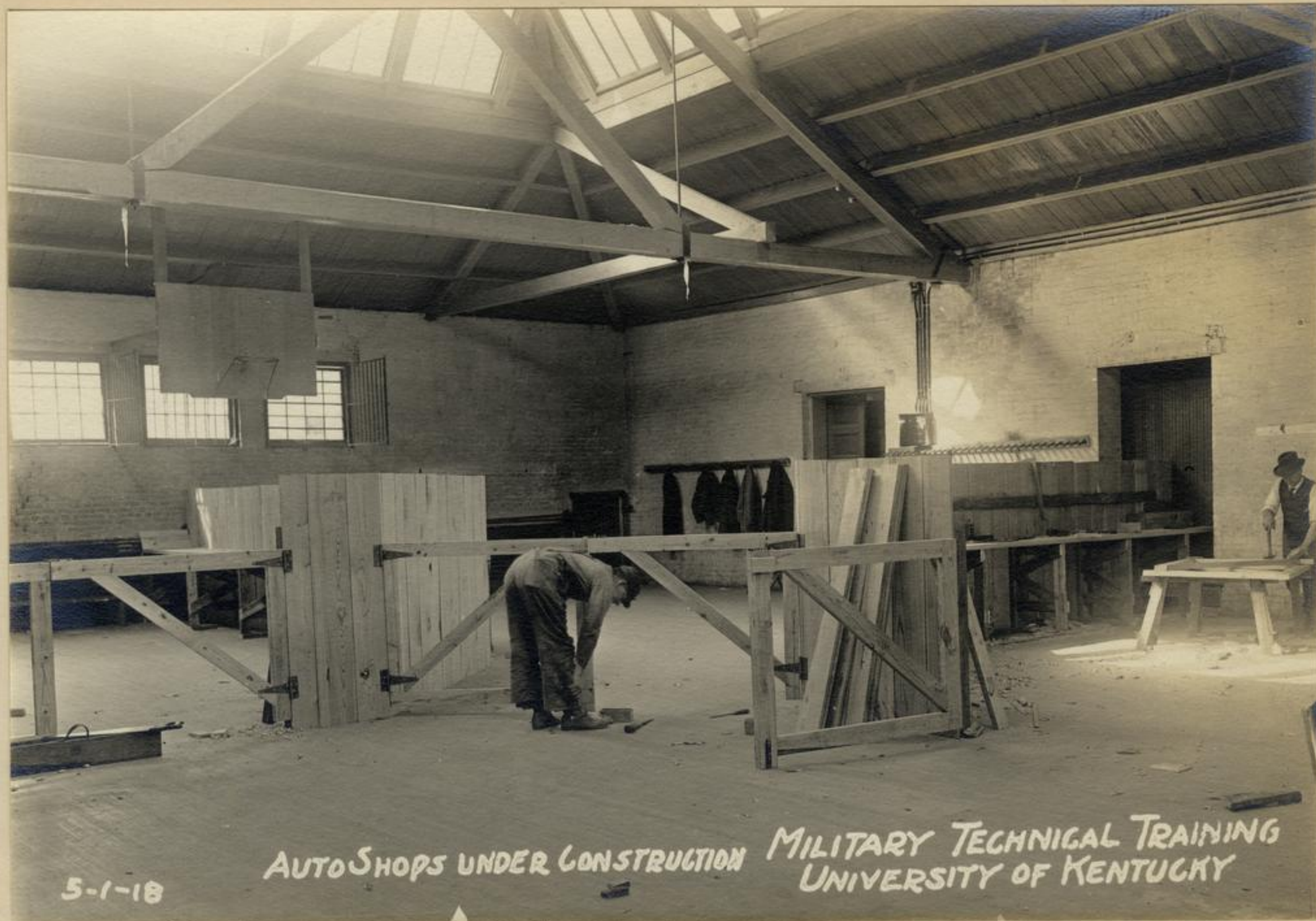
Auto Shops Under Construction, Armory, University of Kentucky Lexington, Kentucky
