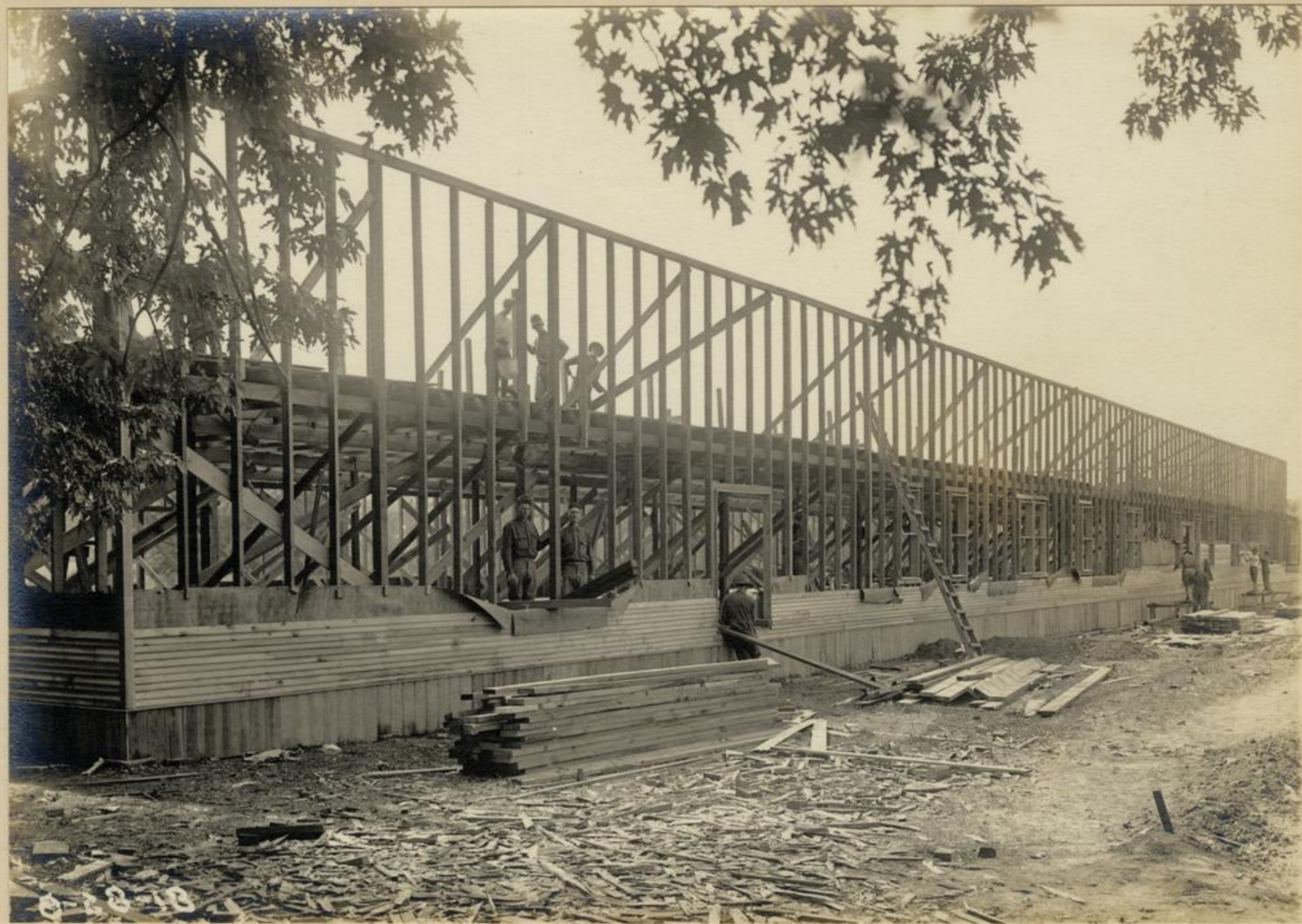
Showing Progress on Second Barracks
