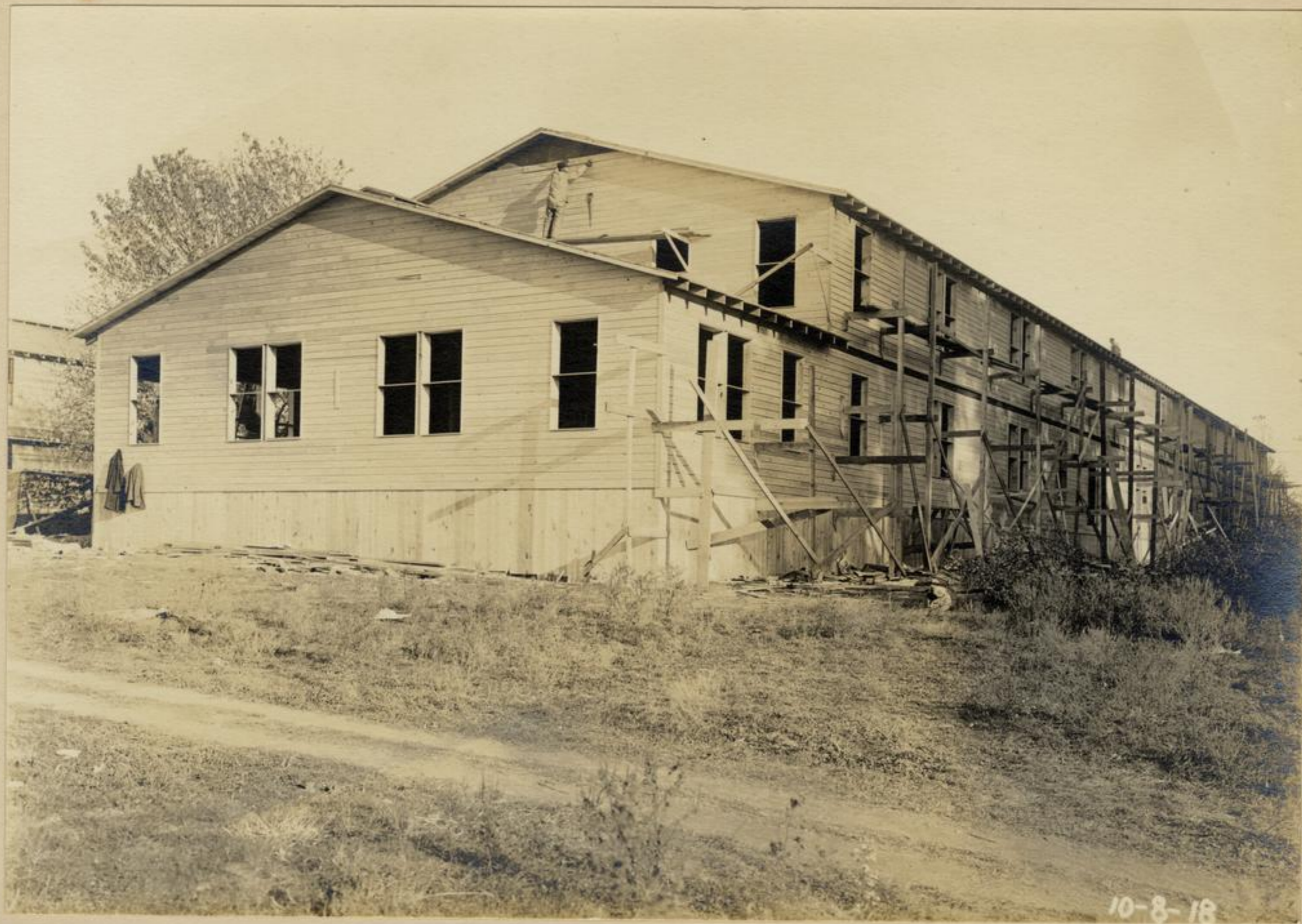
Third Barracks Nearing Completion
