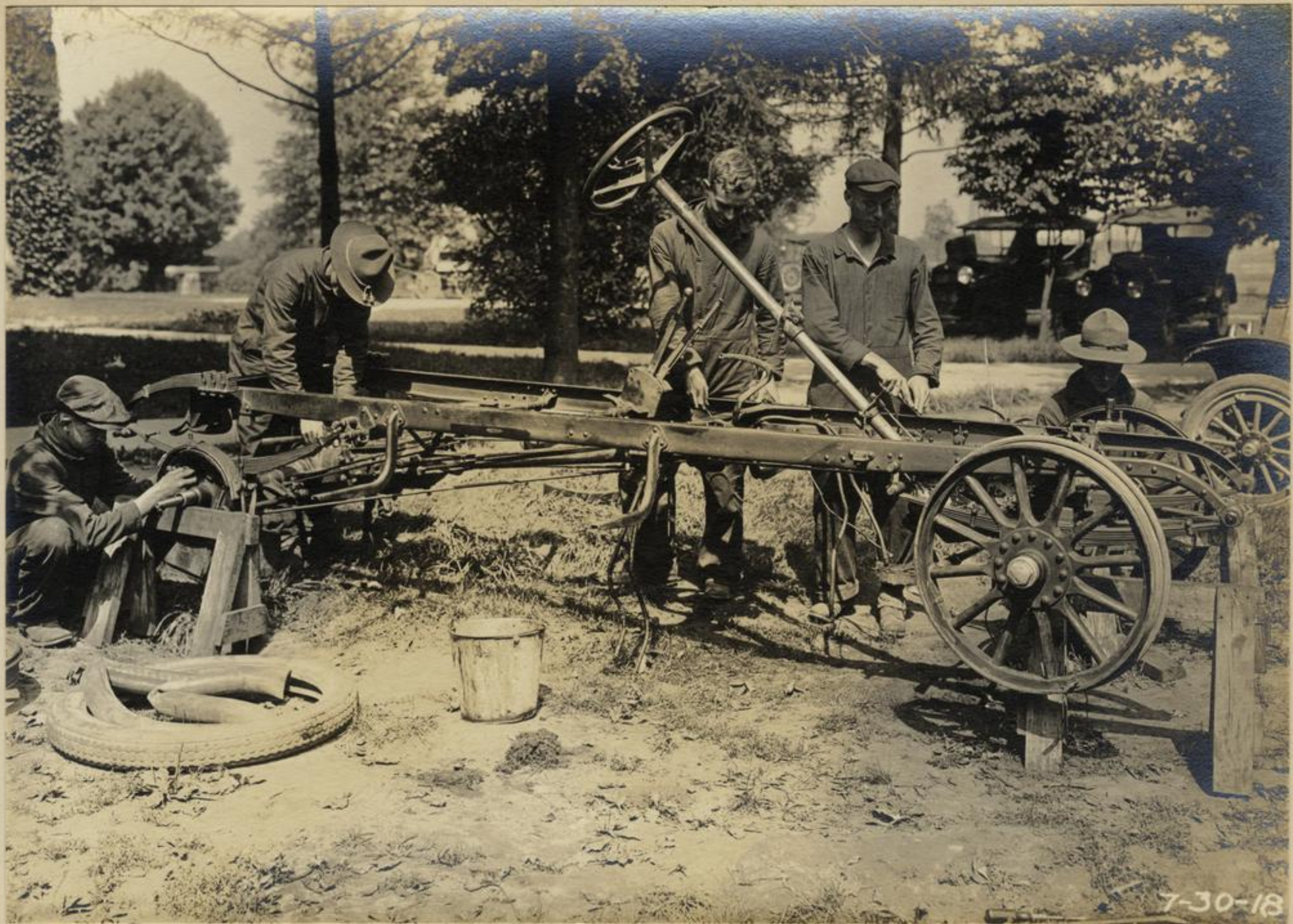
Stripping a Machine Preparatory to Reassembling
