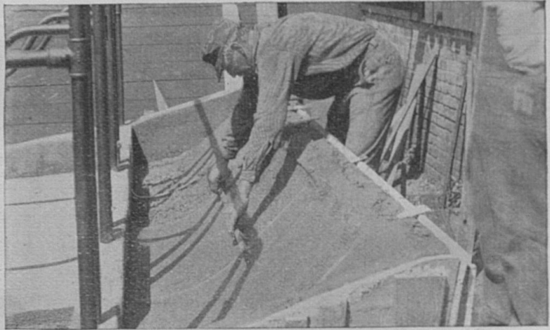
Fig. XI. The manufacturers of barn equipment furnish all templates and information required for constructing the mangers, and instructions should be carefully followed. Picture shows the use of templates for accurately shaping the mangers. Manger surface should then be smoothed with a metal trowel.
