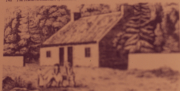
Fig. 127 Double Cottage, Midlothian, 1796. Some stone-faced double front with corrugated half-gabled thatched roof. Although designs of this type were produced and adopted, they appear to have had little effect on the country built stock. The single front plan being more generally adopted even towards the end of the nineteenth century. (Revised, 1880, from Robertson 1796, facing 100)
