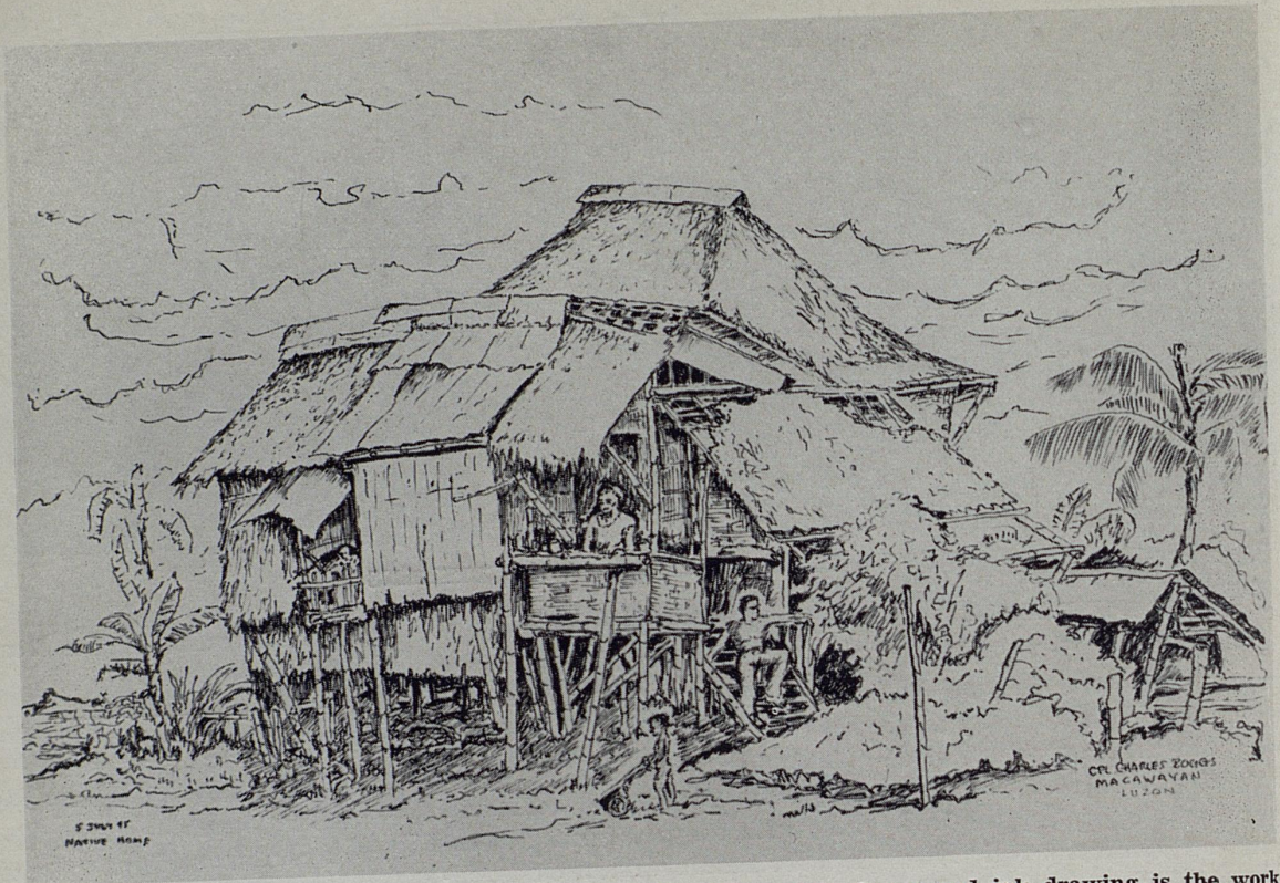
FILIPINO HOME, MACAWAYAN, LUZON —This delicately conceived pen and ink drawing is the work of Corporal Charles G. Boggs. Typical of many homes in the Philippines, it is constructed of nipa with bamboo supports and bamboo floors. Homes are usually raised on stilts to ward off the dampness resulting from the heavy seasonal rains which the Philippines experiences.
