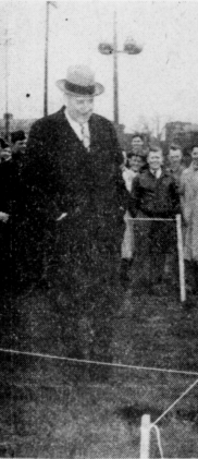
GROUND FORMALLY BROKEN FOR UK FIELD HOUSE—Gov. Simon S. Willis, left, looks on as President Donovan throws a shovel of dirt.
