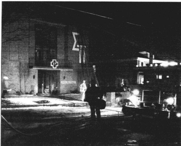
The Sigma Pi fraternity house was burned beyond repair last spring as the result of careless use of a space-heater. No one was seriously injured in the fire.
