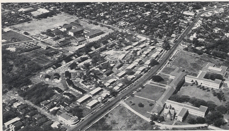
Aerial view of Kamehameha Homes, one of three USHA-aided low-rent housing projects being constructed in Honolulu, T. H. The three projects will rehouse 732 families and destroy an equal number of slum dwellings. Island officials state that behind a
