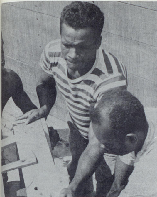
WILLING AND ABLE INDIVIDUALS help load trucks with heavy transformers donated by the people of Kentucky to the people in Santo Domingo de los Colorados.
